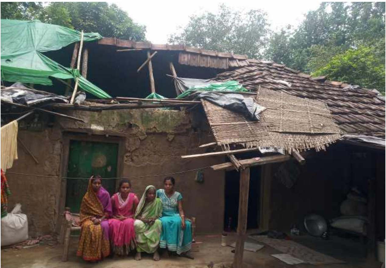
FIGURE 15: DAMAGED HOUSES IN BHADRAK DISTRICT (IMAGE 1 & 2) AND MAYUBHANJ DISTRICT (IMAGE 3)
